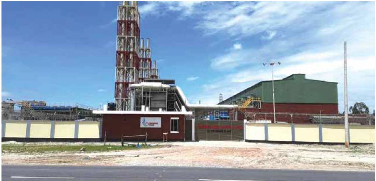
Confidence Power Rangpur Ltd., a 113 MW Power Plant project at Rangpur financed by BDBL
